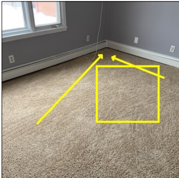
Floor sloped in this direction. Heaving in square. Recommend engineer evaluation. Does not appear to affect foundation.
