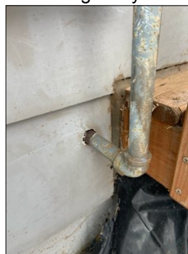
Deck attached directly to home as it should be.
