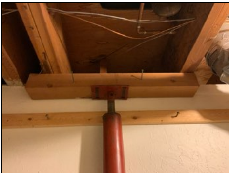
Recommend anchoring all supports.
