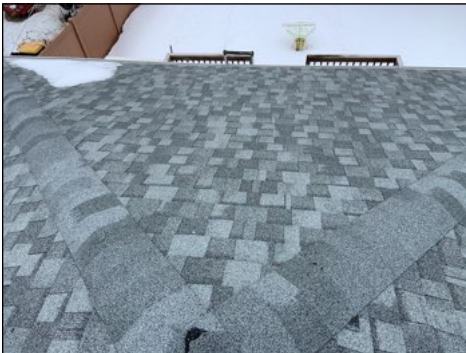
South slope of home.
