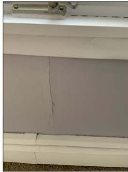
Seam cracks under and above windows and doors. Do not appear structural in nature.
