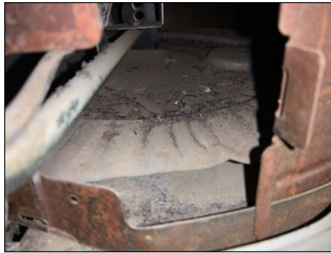
Corrosion in burn chamber.
