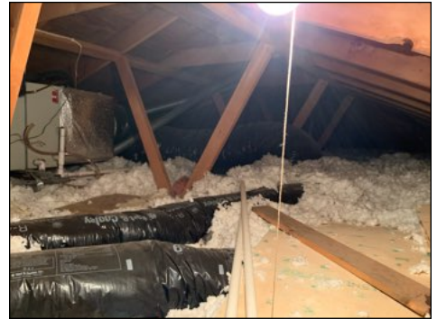
Trampled insulation may contribute to cracking in hallway ceiling below. Recommend releveling insulation.
