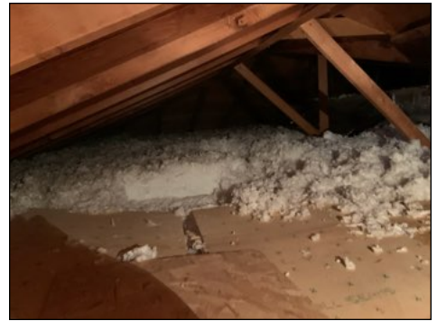
Trampled insulation may contribute to cracking in hallway ceiling below. Recommend releveling insulation.
