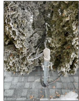
No clearance available for electrical service. 24" is required. Recommend removing trees at rear of home.
