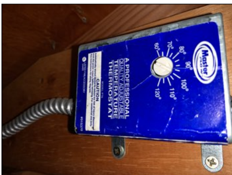
Recommend replacing with combination humidistat and thermostat.
