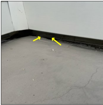
Up to 2" of patch material in downstairs living room subfloor.
