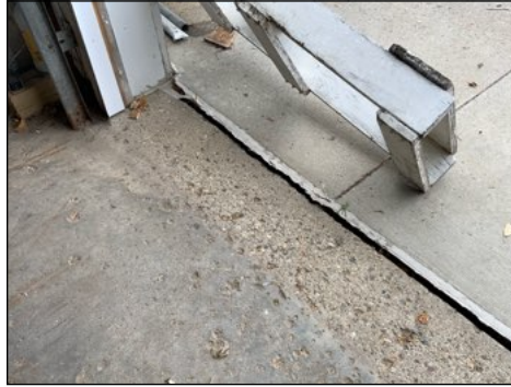
Driveway is heaved compared to garage due to moisture under it. Recommend sealing joint between slabs.
