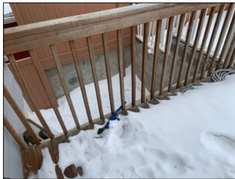
Finish coat degraded. Recommend staining this year.
