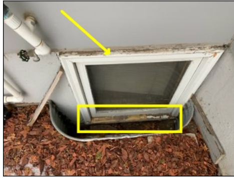
Recommend flashing be installed on top of windows when new siding is installed. Recommend repair of damaged sills, priming and painting.
