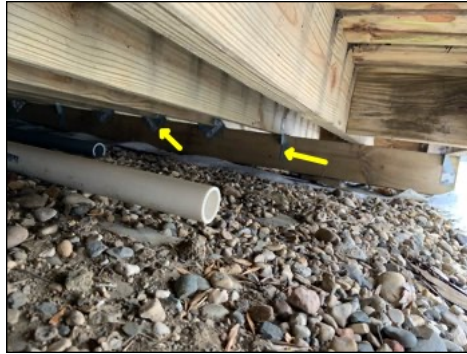
Proper clips installed on girder.
