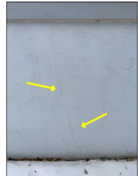
Recommend sealing small crack in north foundation wall.
