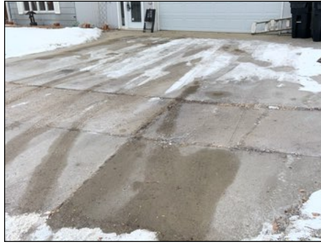
Recommend sealing all cracks and joints with self leveling concrete seal.
