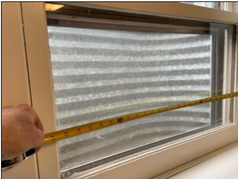
Note all bedroom windows have smaller size openings than modern standards of 5.7SF.
