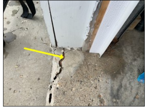
Concrete patch where drive meets garage.
