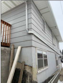
Southwest corner of home.
