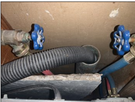
Recommend installing metal braided hoses downstairs.
