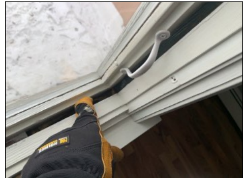
Living room window off hinge, damaged. Recommend repair/replace.
