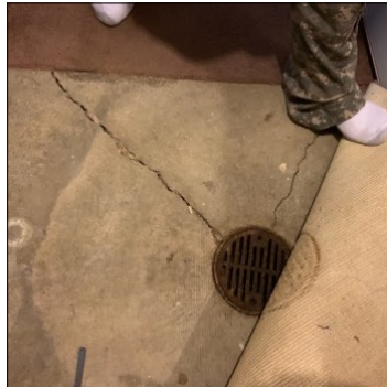
Slight cracking in slab in utility room. Recommend sealing.
