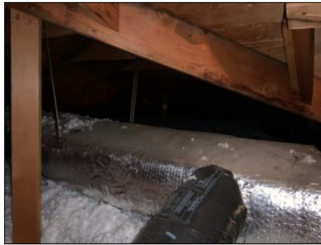
A/C ducting in attic.
