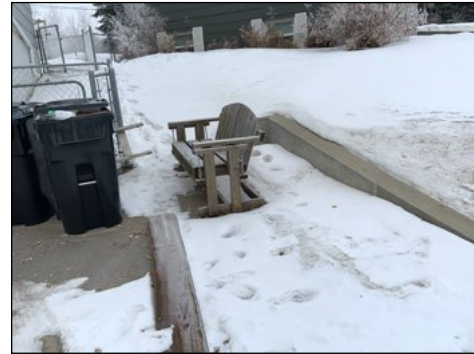
Small retaining wall up front to create a parking area.
