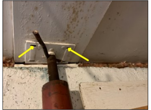
Recommend anchoring all posts.
