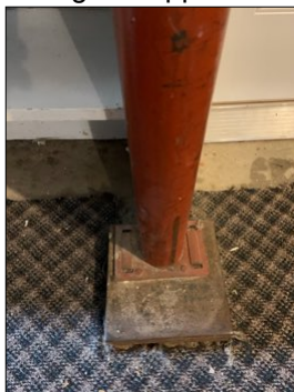
Recommend anchoring all supports.
