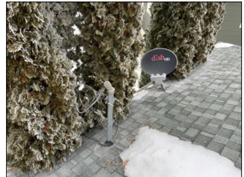
Once tress are removed, debris on shingles won't be an issue.
