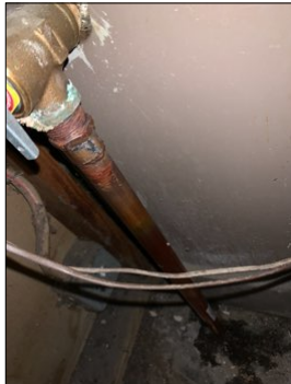
Leaking pressure relief on boiler.
