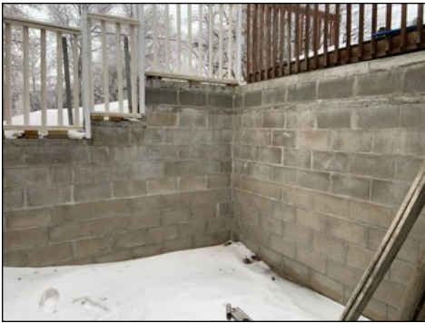
South retaining wall in acceptable condition. Monitor as no weep drains are present.
