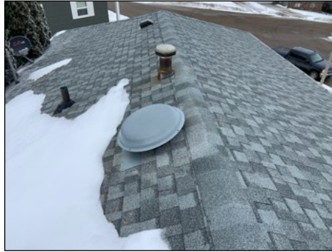
West slope of home. Note attic vent fan.
