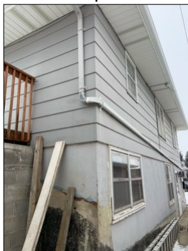
Note north gutter diversion not hooked up.
