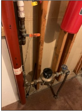
Main water shut off in downstairs utility room.
