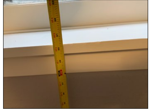
Note all bedrooms have sills that higher than modern standard of 44" recommend advising tenants to place furniture under windows.
