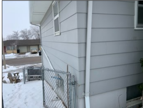
Northwest corner of home.
