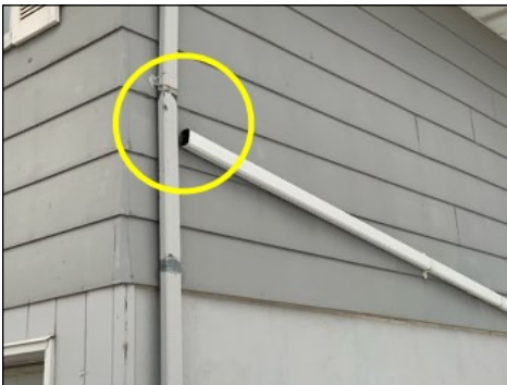
Note north gutter diversion not hooked up.
