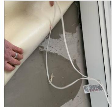
Cracking in recent floor leveling indicates pressure from below.
