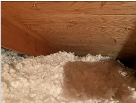
No baffles present. Ventilation appears adequate.
