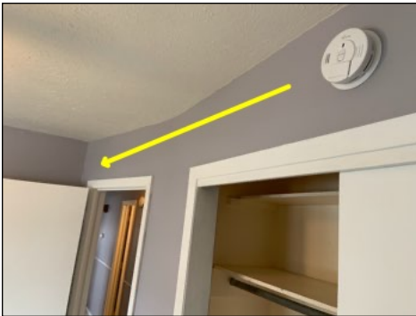
Recommend ceiling mounting detectors to main entrance of rooms.
